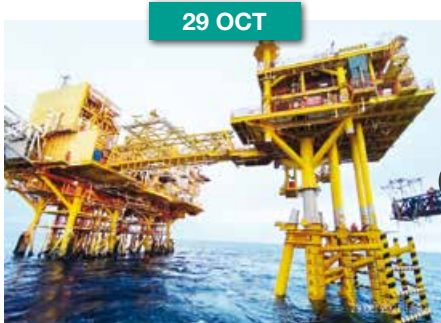
Completion of the installation of Bekok Oil Project AA (Bekok AA)
