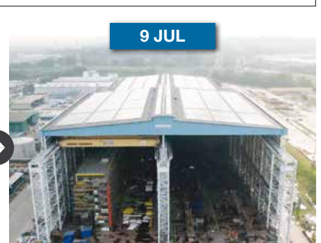
MHB powers up operation with Solar Panels which represents Malaysia's Largest Rooftop Solar Panels installed in a single compound
