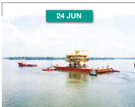
Sail away of WHP Topside of Kasawari Gas Development Project
