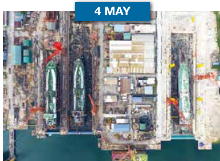
Dry Docks at full capacity with 3 LNGCs
