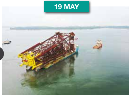
Sail away of WHP Jacket for Kasawari Gas Development Project
