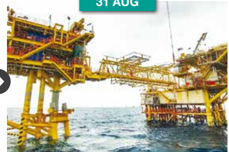
Completion of the Installation of Bekok Oil Project BB (Bekok BB)
