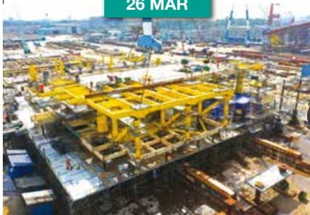
Achievement of 5 Million Safe Man-days for Kasawari Gas Development Project
